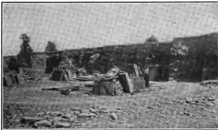
FIG. 1259. — Stewart flagstone quarry in upper Hamilton formation north of Rensselaerville, N. Y. The flagstones are obtained from the massive layers in the bottom of the quarry ( 4\frac{1}{2} to 6 ft.) above which lie shales with Hamilton fossils, capped by glacial material. (Photo by C. S. Prosser; courtesy N. Y. State Museum, John M. Clarke, Director.)
